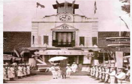
Bangunan Mahkamah • Court House building, 1941
