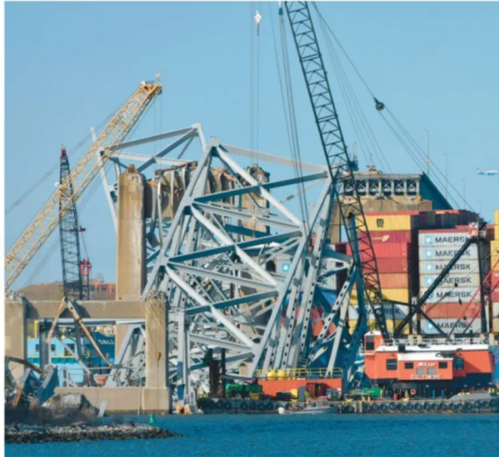
The wreckage of the Francis Scott Key Bridge and the container ship Dali rest against each other in the Patapsco River after the ship struck the bridge on March 26, causing its collapse. AMY DAVIS/STAFF
